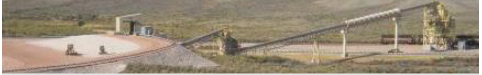
The completed Transloading System allows trucks to dump with passive dust control, just in time delivered via an apron feeder and cleaning screen, to the loading bins above the new tracks. The conveyor tube which crosses the highway is the first of its kind in the State of Montana. The system is automated to regulate speed proportional to the rate of railcar loading, thus minimizing the need for surge bin capacity.
