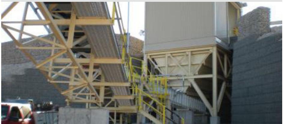
Hilfiger systems were used with the quarry's native rock to establish retaining walls at the truck dump and haul road access area.
