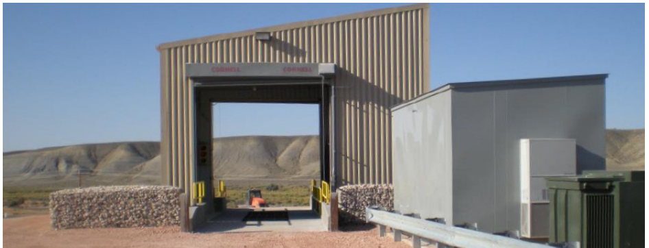
Hilfiger systems were used with the quarry's native rock to establish retaining walls at the truck dump and haul road access area.
