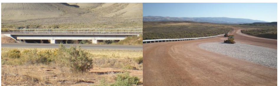
Benetech designed & constructed viaducts, a rail bridge, and approximately three miles of spurs and switches. The most challenging task was designing around landscape constraints, logistics, and cost. The design/construction required submittal of permits with EPA, State, County and Army Corps. Land ownership was also a design issue.
