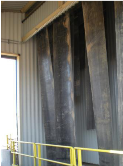
Passive dust hood channels air around and back through hanging belts to slow air velocity and impinge/drop out dust.
