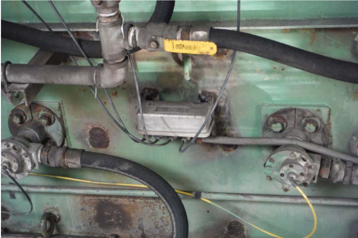
Pilot Valve Box Location and 1/4" Tube
