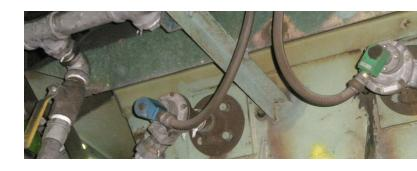
Electronic controls trigger the Clean Sweep nozzles, firing in a predetermined order.
